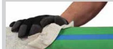
Remove standing dirt and oil using an isopropyl alcohol-based cleaner (70% by volume or greater). Dirty pipe will not form proper beads during fusion. Be careful not to wipe off the printed label.
