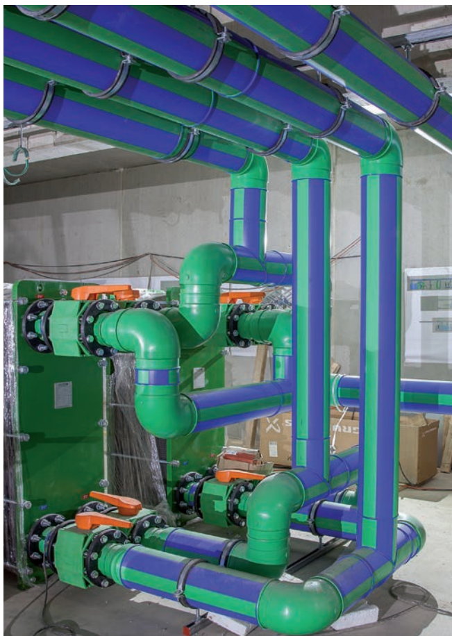
Commissioning of the system for process cooling
