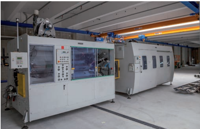
Week 27: Installation of the first plant in the new building
