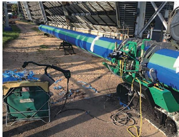
After completing Aquatherm's factory certification training (necessary to enact Aquatherm's 10-year, multimillion dollar warranty, along with a thorough pressure test), the installation team moved the fusion process along quickly and smoothly using a McElroy PolyHorse pipe-handling system. The installation was completed within 24 hours.
