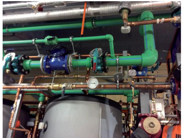
A very well detailed domestic hot water plant room using aquatherm pipes.
