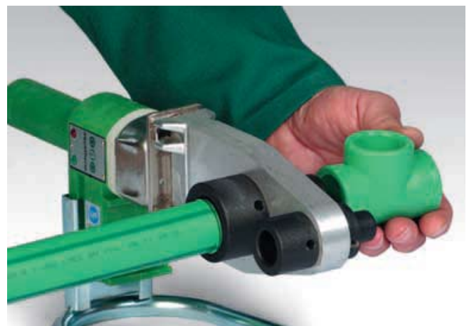
Heating-up of pipe and fitting
