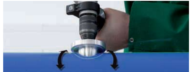
Removal of the oxgen barrier layer from the climatherm OT-pipe
