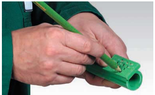
Marking of the welding depth
